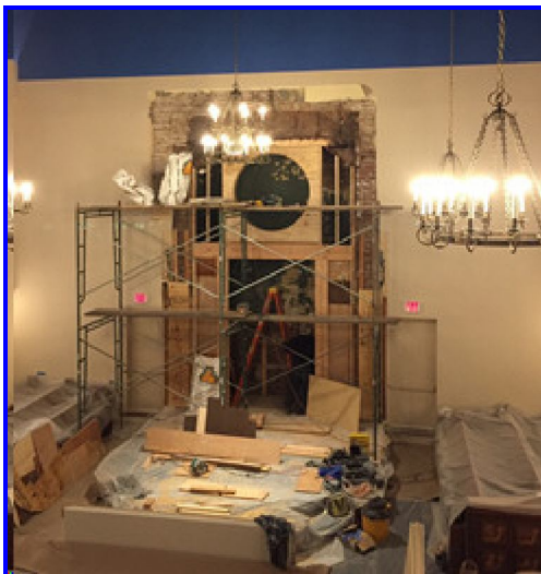
Ark wall under construction
